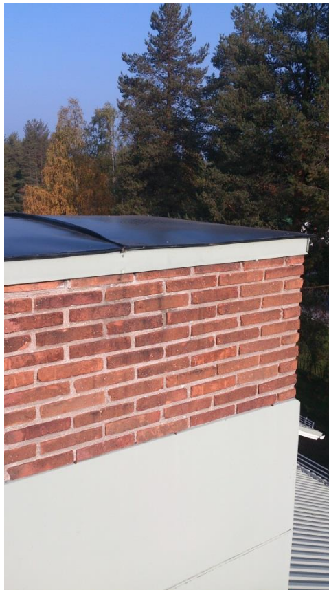
Figure 3.22 The surrounding environment of station Vidsele, and the antenna is mounted on the side of the chimney (The photo is provided by Lantmäteriet).
