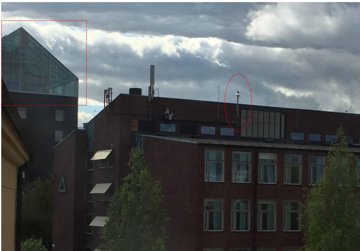
Figure 3.1 Photo for the mounted antenna of station KTH.
