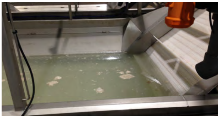
c) The waste is collected by the source, and the water is collected underneath the sieves and sent for further treatment.
