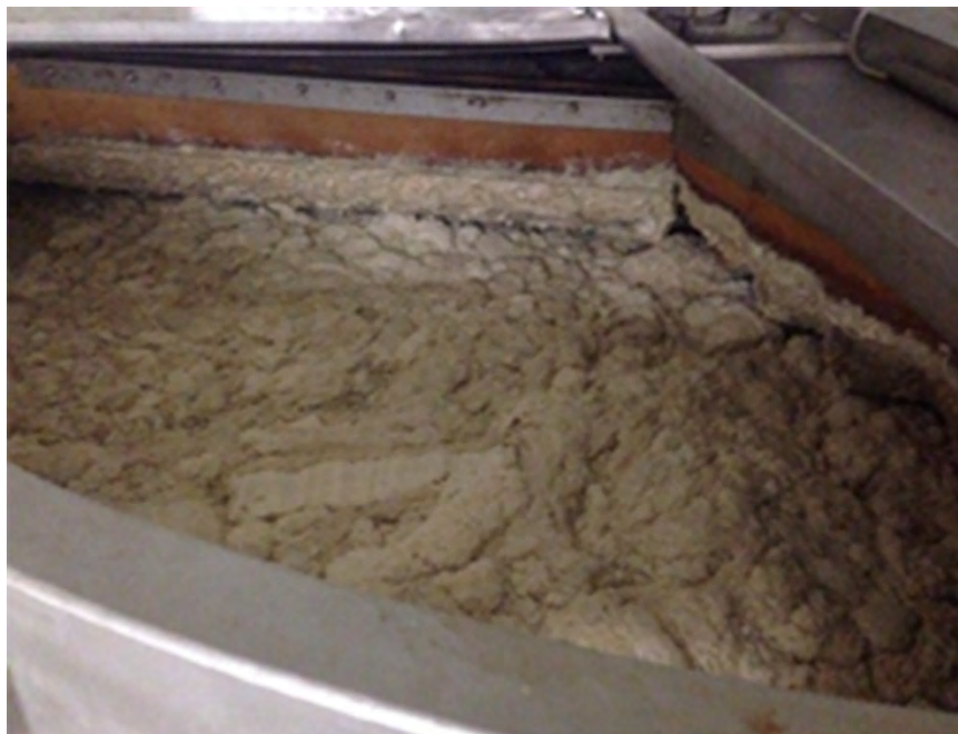
Figure 21. A DAF unit is used to remove fat and oil from the water; here the fat is seen on the surface of the flotation unit
