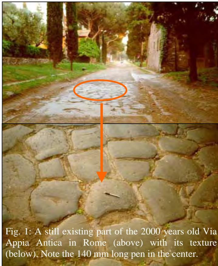
Fig. 1: A still existing part of the 2000 years old Via Appia Antica in Rome (above) with its texture (below). Note the 140 mm long pen in the center.
