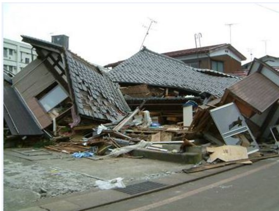
Figure 1. Damaged wood frame houses from Niigata prefecture in Japan, Oct. 2004, magnitude 6.8 on Richter scale [14].
