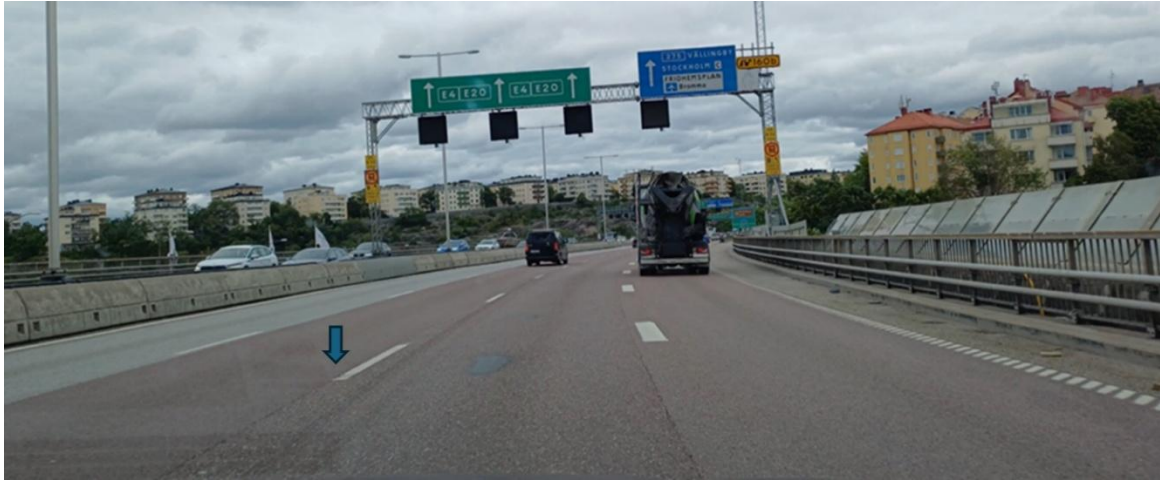
Figure 13: Road area at the beginning of the exit to Lilla Essingen island. The pond is situated below this part of the bridge. The blue arrow indicates the wear of the lane line. On the right-hand side, the so-called stair-flex line is visible.
