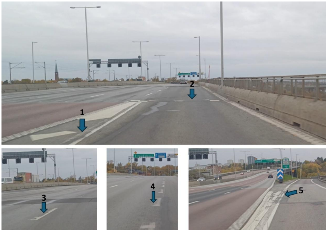
Figure 14: Road marking wear at the entry (1, 2) on the Gröndal bridge (3, 4) and the exit (5) to the district Gröndal. These markings are on vehicles crossing areas with obvious wear and possible release of paint-borne microplastics.
