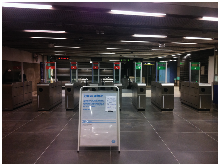
Figure 1. The electronic gate under installation in Stadion metro station during 2015.
