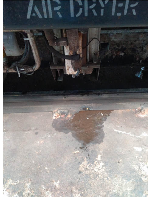
Figure 1: An air dryer ejecting moisture. Unless specified otherwise, all photos by the author.
