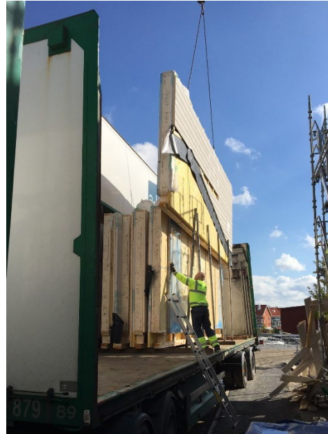
Figure 10: Modules designed for efficient transport: planar wall elements. Photo: Derome.
