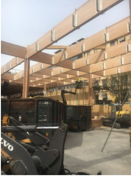
Figure 6: Bolted connections could be undone. Photo Andres Zabala Mejia.
