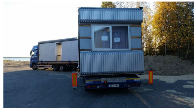
Figure 11: Modules designed for efficient transport: volumetric modules. Two modules can be transported with one vehicle. Photo: Masonite Beams.
