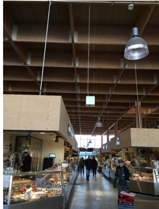
Figure 2: A hall with post and beam structure, that first served as a temporary market hall and later became a sports hall. The photo shows the hall in its first use. Photo: Ylva Sandin
