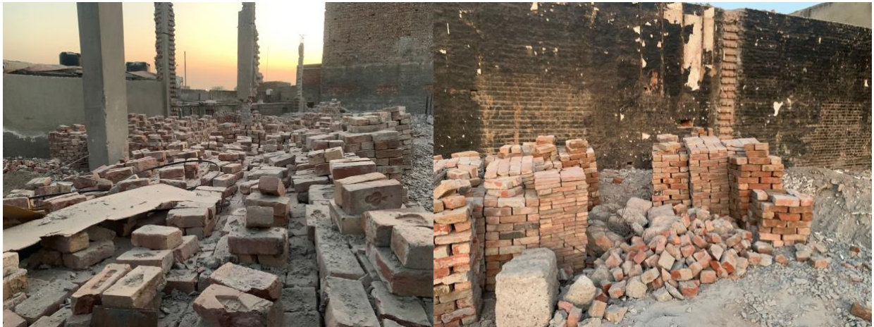
Figure 19 After cleaning of bricks – Ref; Author
