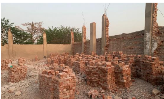
Figure 20 Sorted and ready to transport Reclaimed bricks – Ref, Author.
