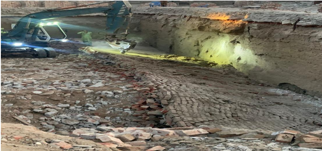
Figure 17 Extraction of bricks by using machinery. Reference, Author
