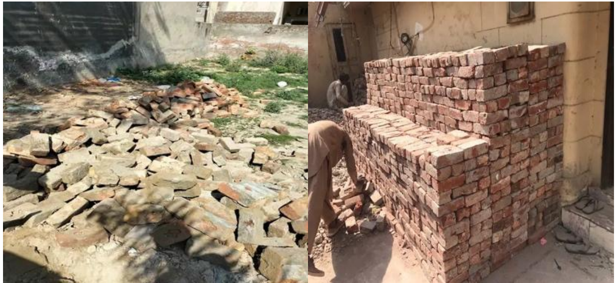
Figure 11 Extraction and storing of reclaimed brick – Ref; Author.
