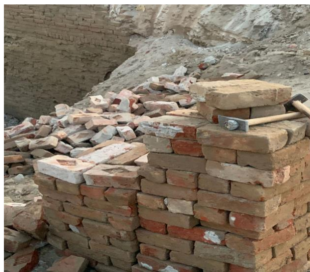
Figure 18 Cleaning bricks by using a chisel hammer - Ref: Author
