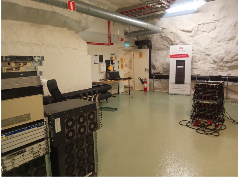
Figure 3. Disorder at HE2 in the process of dismantling.
