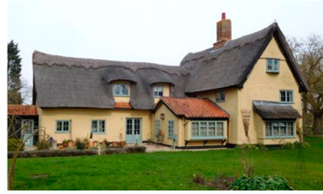
Figure 2. South, elevation. Source: Author's own, 2017.
