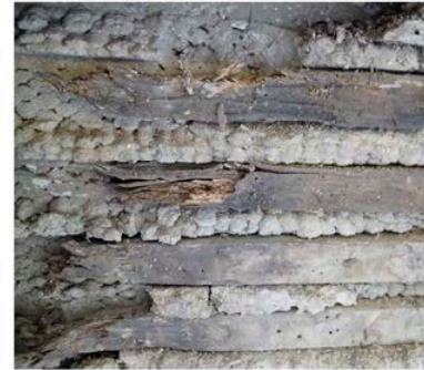
Figure 5. Internal face of cement render. Source: Author's own, 2017.
