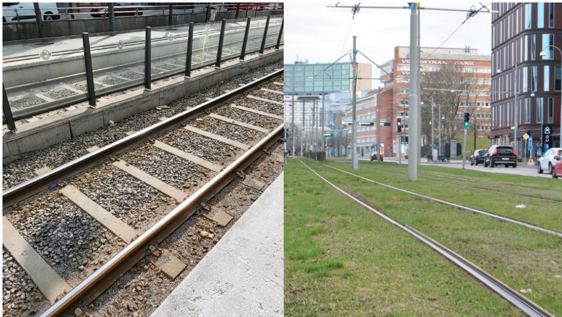
Figure. 1. Macadam track in Hammarby Sjöstad, Stockholm (left), and grass track in Ullevi, Gothenburg (right). Source: Author’s own pictures.
