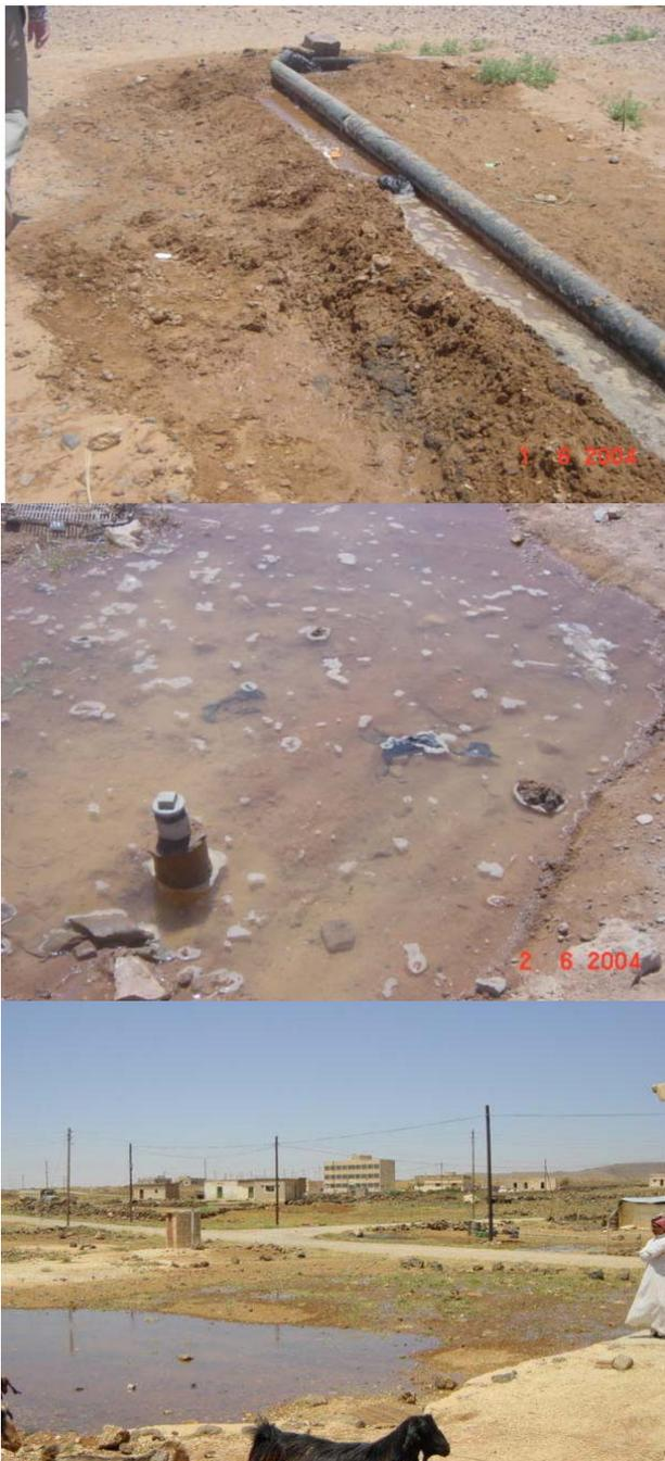
**Figure 7.** Examples of technical losses: up—broken pipe; middle—leaking pipe; down—breaking pipe to supply water to livestock.
