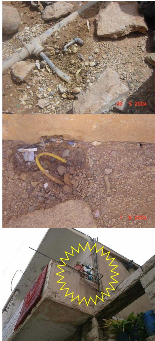
**Figure 8.** Examples of administrative loss in Mafraq: up—the meter is removed and replaced by a T-joint; middle—pipe connection passing the meter; down—connection to supply the housing unit before the meter.
