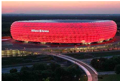
Figure 1.2: Inflated membrane structure, Allianz Arena stadium, Munich, Germany ( https://www.allianz-arena.de )
