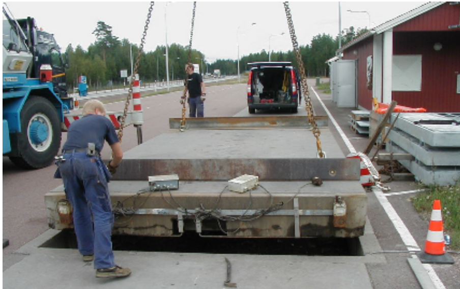
Figure 3.2: Installation of the weighing machine [13]
