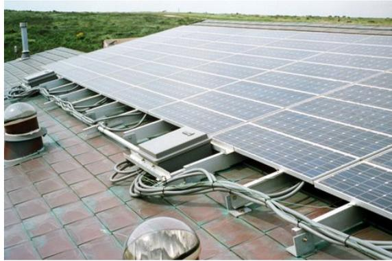
*Illustration 10: BoS components. Cabling, inverter (with case) and mounting frame.*
