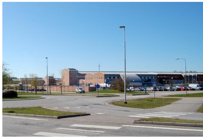
Figure 15 Ericsson R&D base in Linköping, (source - authors picture)
