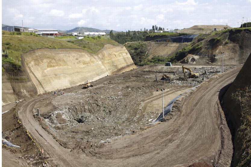
Figure 2: Landfill site under construction (taken from elements.geoscienceworld.org ).
