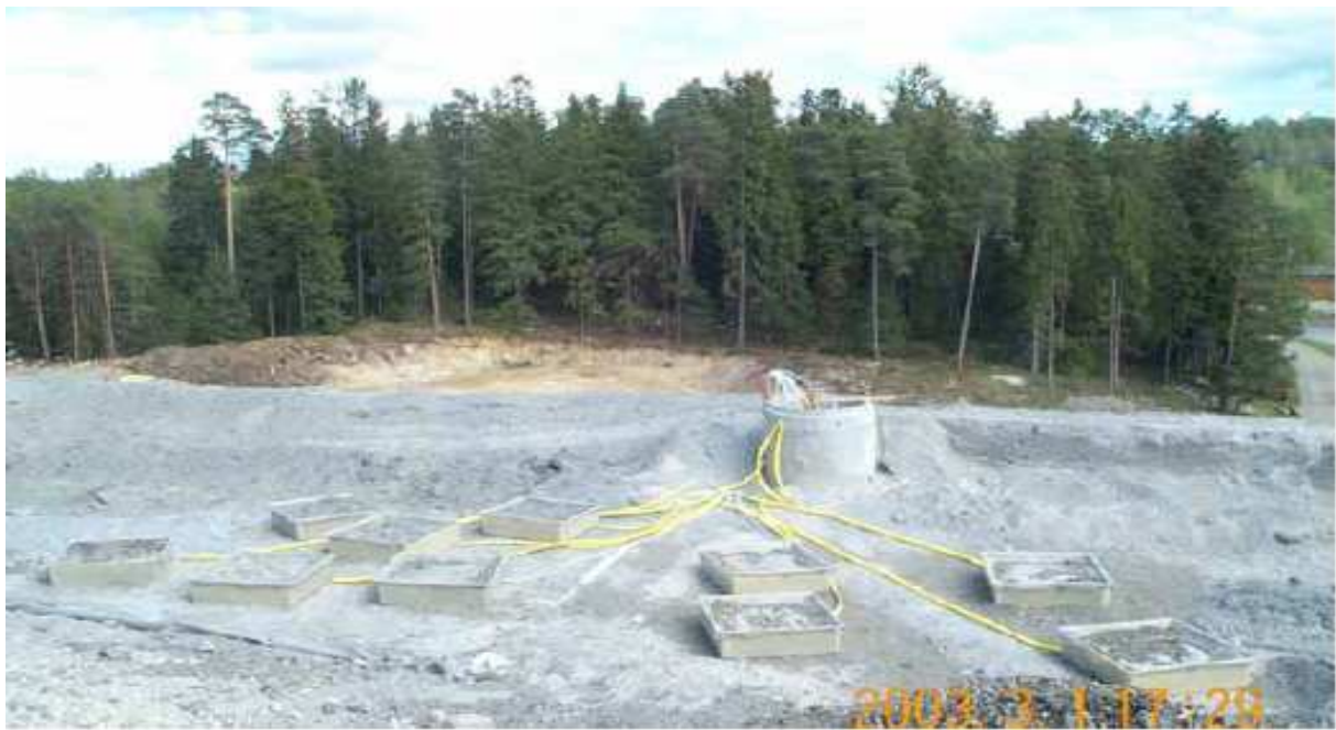
Appendix fig. 8 Installation of lysimeters (Tham & Andreas, 2008).
