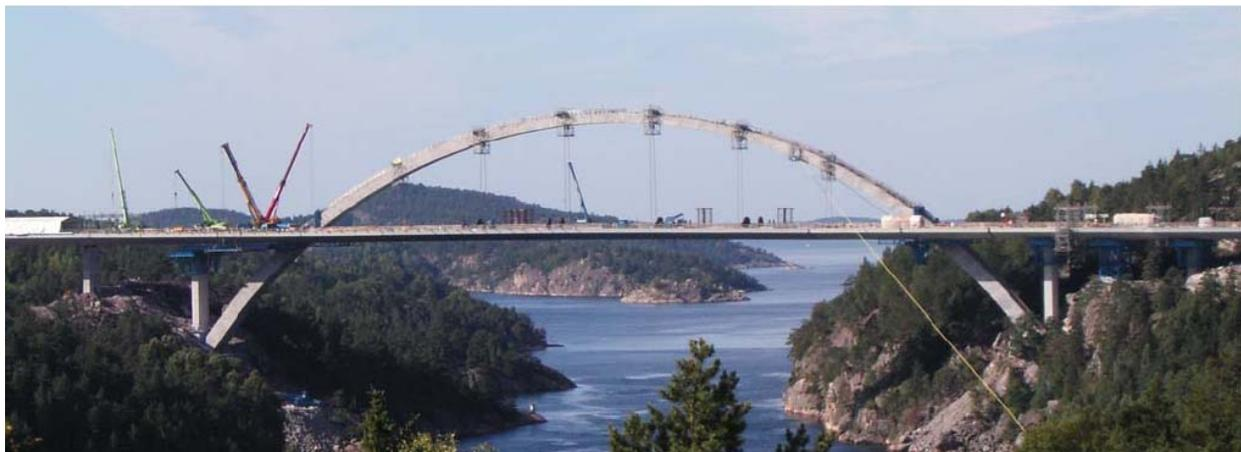
Fig.2 A photograph of the bridge during construction. The temporary towers (can be seen at both arch bases) have not yet been completely removed.
