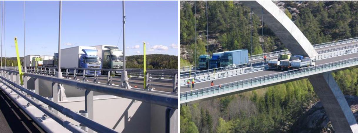
Fig.4 Loading patterns C with 8 lorries (left photo) and E with 6 lorries (right photo)
