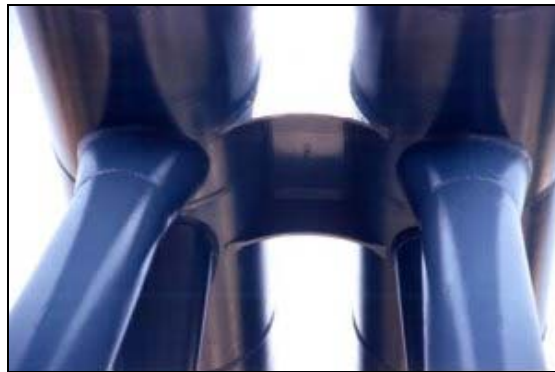
Figure 109: Picture of the union between the arch and triangulation tubes
