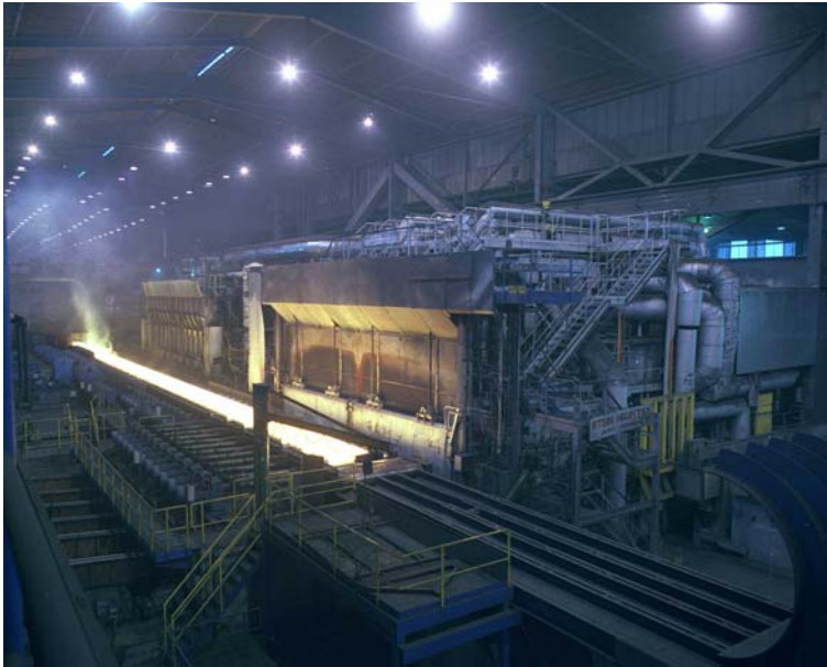
Figure 4: Hot rolling at Outokumpu Stainless Avesta works. The roughing mill is located at the far left. Two walking-beam reheating furnaces are seen to the right.
