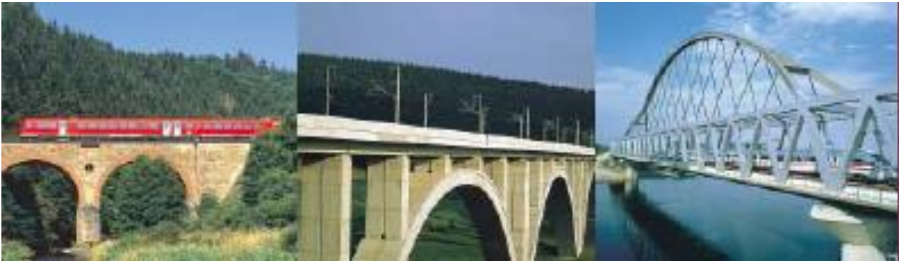
Figure 1. Three types of existing railway bridges being studied: Masonry Arches, Steel Beams supported by Reinforced Concrete Arches and a Steel Truss carried by a Steel Arch.
