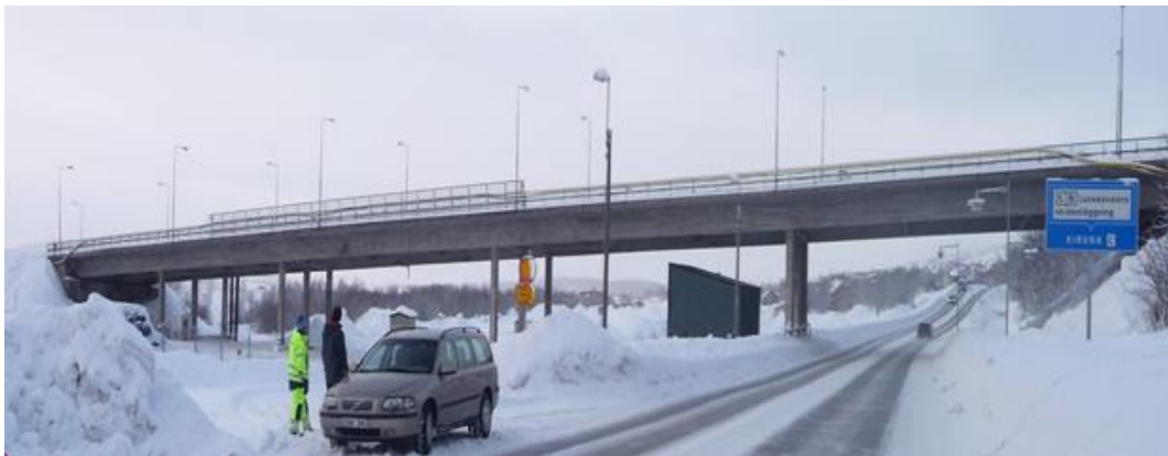
Figure 1. Kiruna Bridge constructed in 1959, Nilimaa et al. [3]
