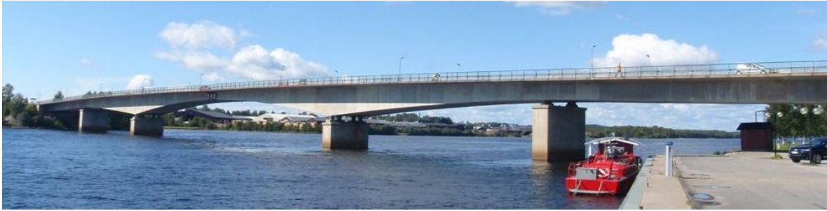
Figure 7. Bridge over Kalix River in Kalix, view towards south.
