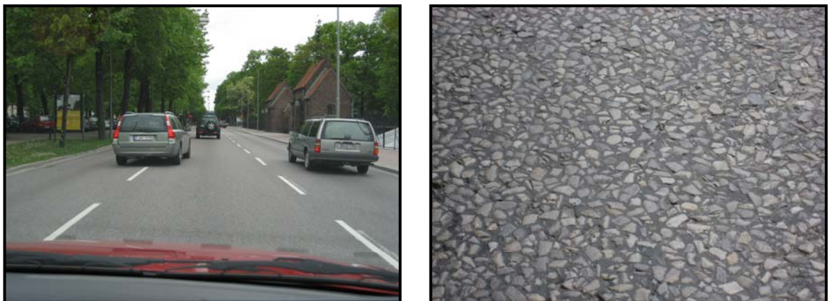
Fig. 4.1 and 4.2. Test conditions and zoom of the asphalt
