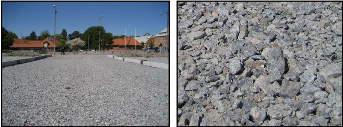
Fig. 4.9 and 4.10. Gravel surface of the test and zoom of the gravel
