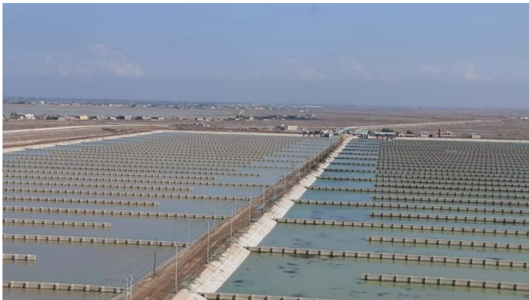
Figure 5: General view of R0 reservoir. (Source: [1]).
