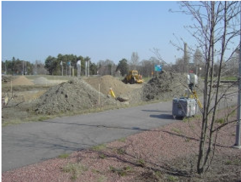
Figure 7: picture of the piles
