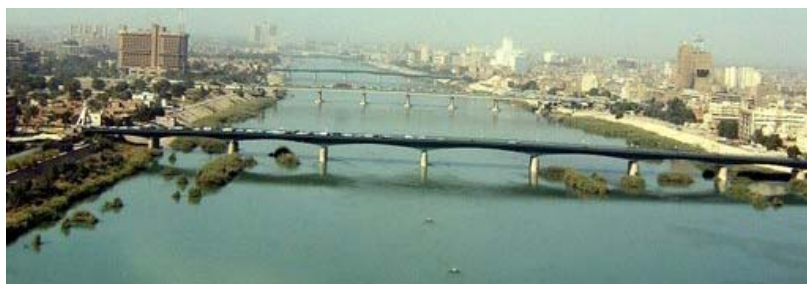
Figure 4: Small growing islands at Jumhuriyah Bridge location.
